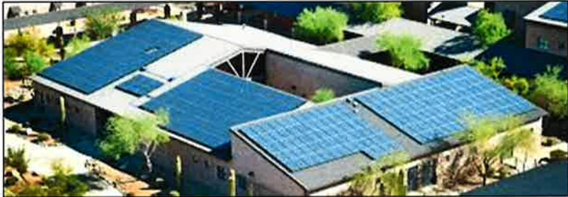
Renewable Energy – Roof Solar Paneling
