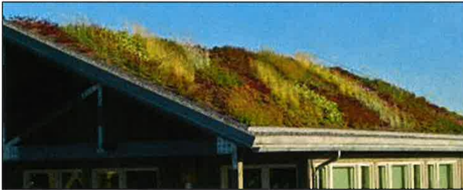
Green Roofs to Reduce Storm Water Runoff, Reduce Building Energy Use and Promote Cleaner Air
