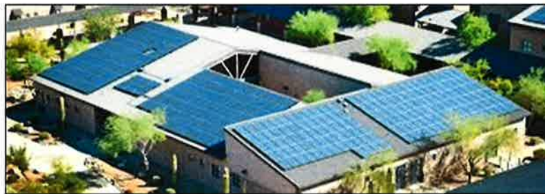
Renewable Energy – Roof Solar Paneling
