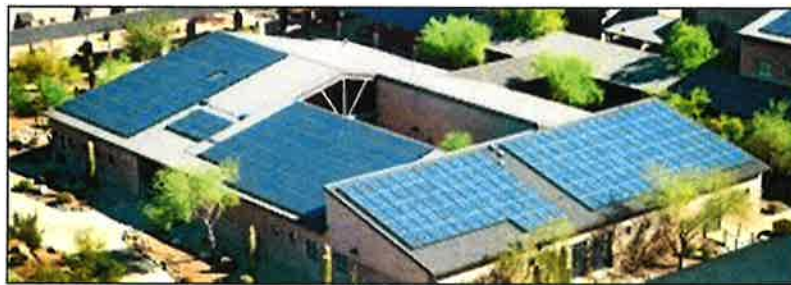
Renewable Energy – Roof Solar Paneling
