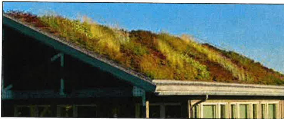
Green Roofs to Reduce Storm Water Runoff, Reduce Building Energy Use and Promote Cleaner Air
