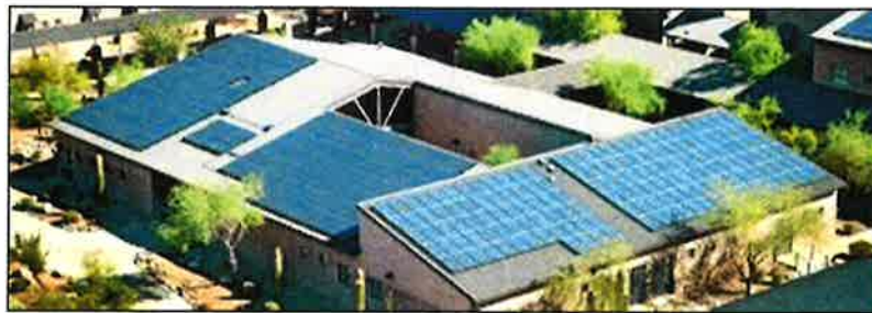
Renewable Energy – Roof Solar Paneling
