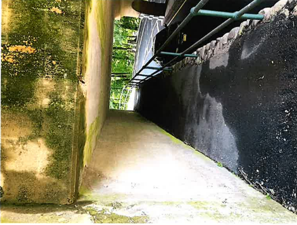
PHOTO 4 – WALKWAY UNDER TRESTLE
