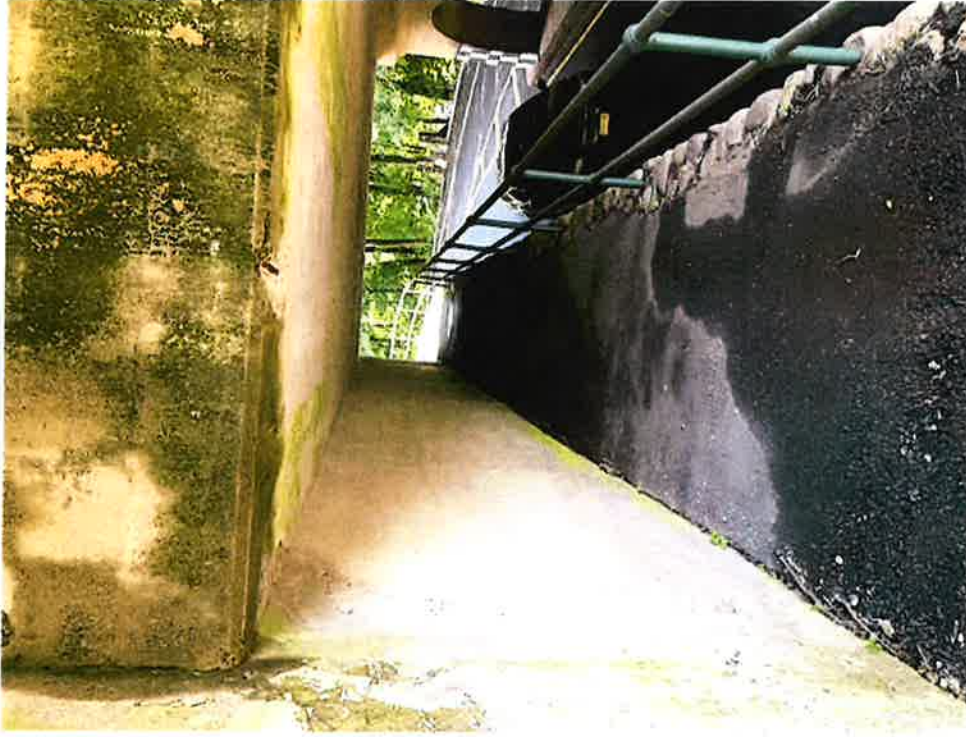
PHOTO 4 – WALKWAY UNDER TRESTLE
