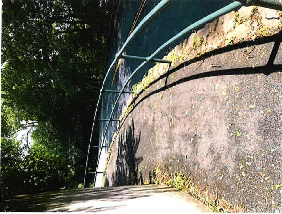
PHOTO 2 – WALKWAY ON SOUTH SIDE OF TRESTLE
