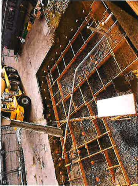
Footings for Back Addition
