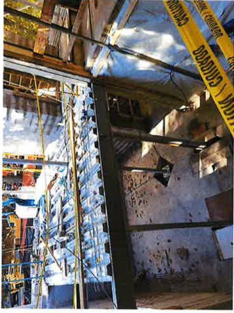
Steel Supports and Decking at Front Addition
