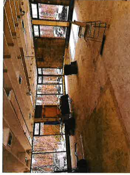
Demolition of Former Board of Education Space
